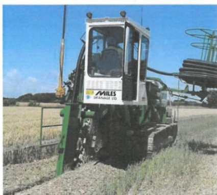
Figure 31. Installing land drains with laser gradient control
