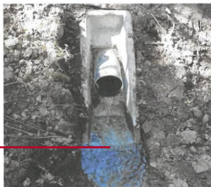
Figure 38. Precast concrete headwall (type K)
