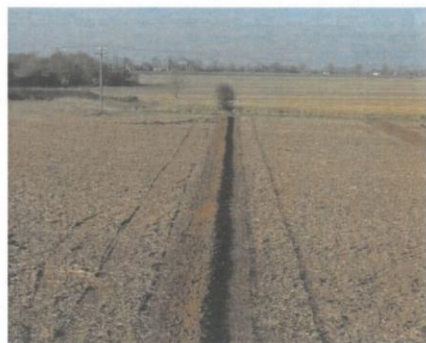
Figure 29. Recently installed drains
