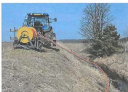
Figure 23. Drain jetting
