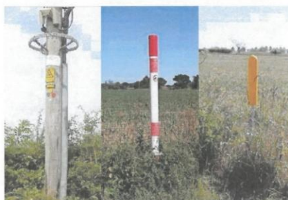
Figure 18. Signs indicating potential underground hazards
