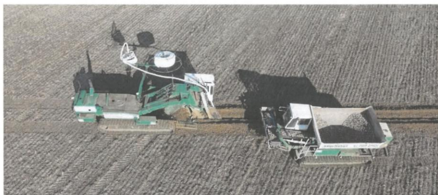
Figure 28. Installing land drains and stone backfill
