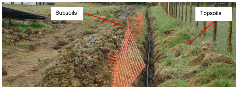
Photo 26: Subsoils Dug out of the Trench
