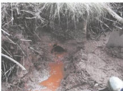
Figure 21. A blocked outfall can often be cleared in a matter of minutes with a spade
