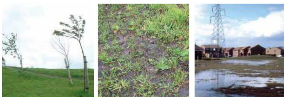
The symptoms of over-compaction of soil on the amenity areas of new housing estates: struggling trees; poor grass growth; and surface ponding after heavy rain.
