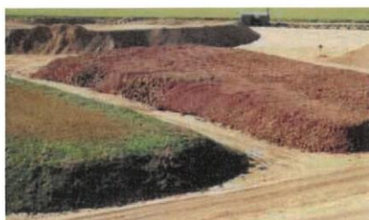
Clearly defined stockpiling of different soil materials
