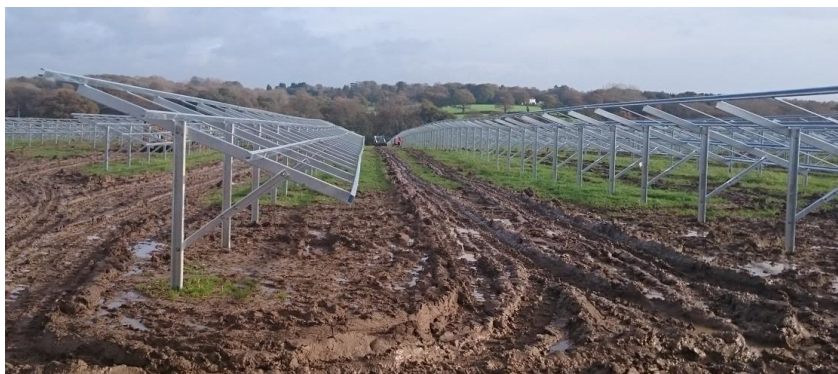
Photos 5 and 6: Inter-row Localised Soil Disturbance and Subsequent Restoration
