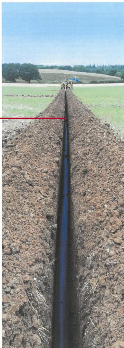
Figure 32. Install drains at an appropriate depth and constant gradient (fall)
