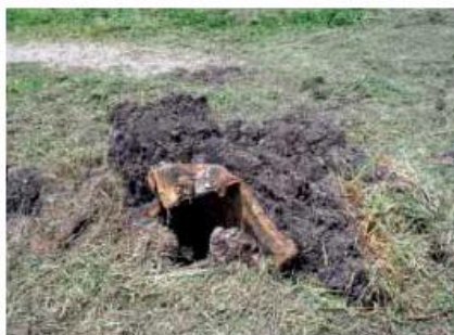
One of many items of debris encountered in the imported topsoil during remedial works
