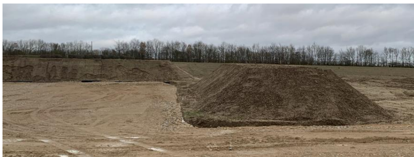
Photo 14: Topsoil Storage Example
