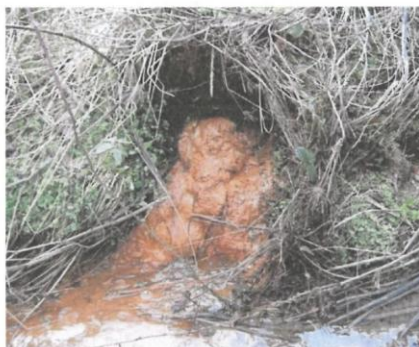
Figure 24. Drainage outfall blocked by ochre
